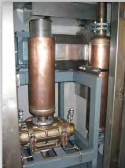
Air-scour Blower in Corrosion-resistant Materials
