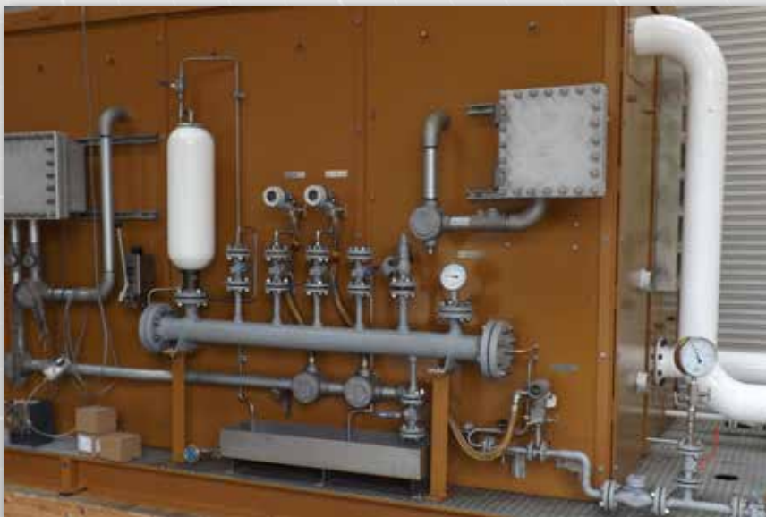
Seal Oil Supply System to API Standard 682, Plan 53B
