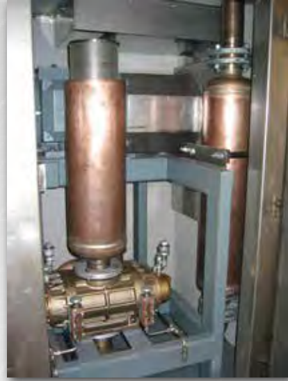
Air-scour Blower in Corrosion-resistant Materials
